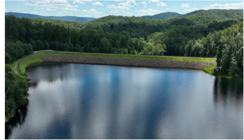
Ragged Mountain Reservoir and Dam
