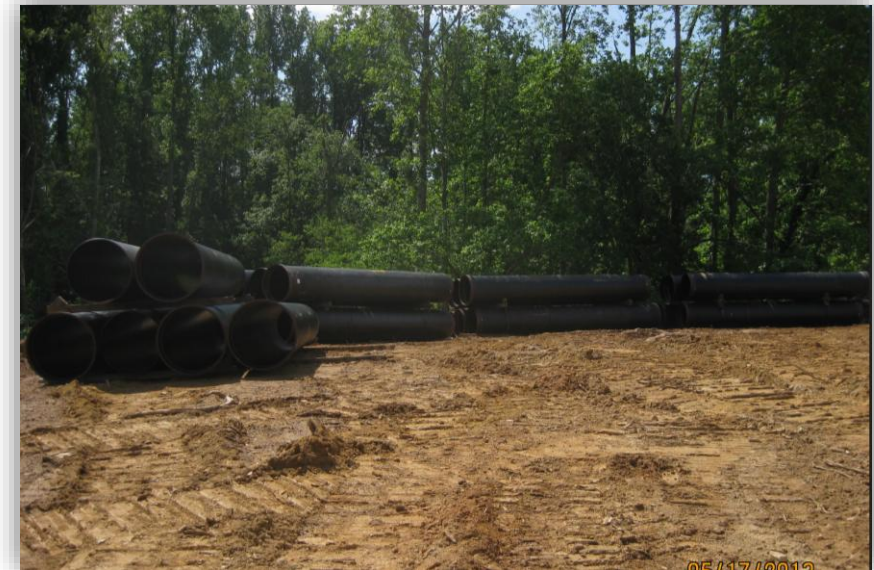
New Ductile Iron Pipe 2013
